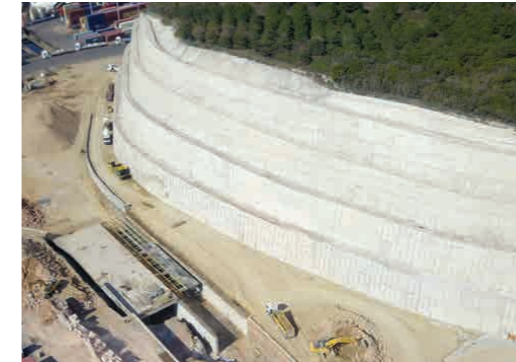
Earthwork and Retaining Wall Construction
